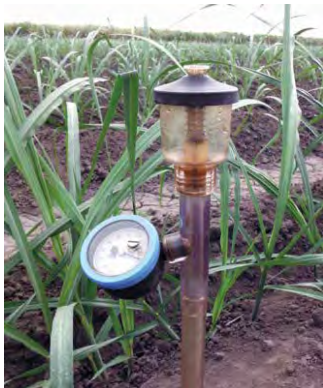
Above: Tensiometer installed in a field.
