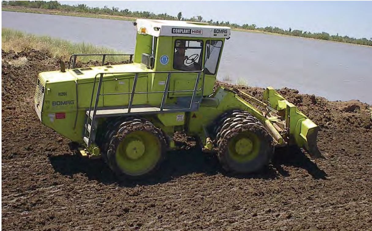
Figure 7.2. Compacting earth fill placed in an embankment breach
