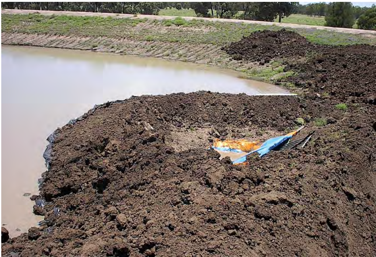
Figure 7.1. An embankment (and water) saved by placing a tarpaulin over the breach, followed by an earthen coffer dam.
