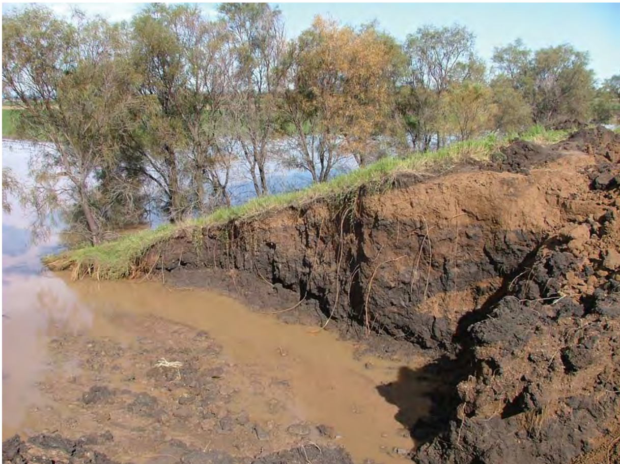
Figure 5.5 Tree growth near storage embankments should be discouraged
