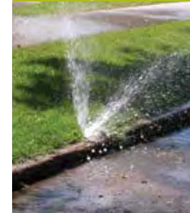
Inundated Water Caused by Broken Irrigation Pipes
