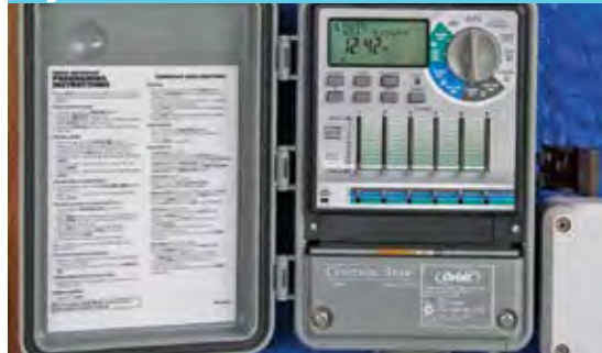
Irrigation Controller
