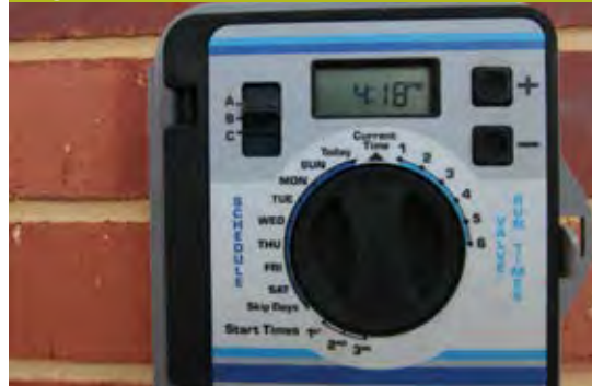
Irrigation Controller
